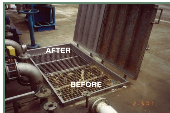
Cleaning of waste water pits using Triple7 products
